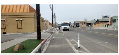
A high-quality bicycle facility on 5th Street will require attention to snow removal protocol and adjustments to parking spaces which are too close to driveways for sufficient sight distances. Parking adjacent to a separated bike lane pushes vehicles further into the roadway, creating sight distance issues for drivers entering and exiting a driveway. To provide adequate sight distance, parking should be prohibited at least 20 ft from the edge of a driveway, on both sides.
